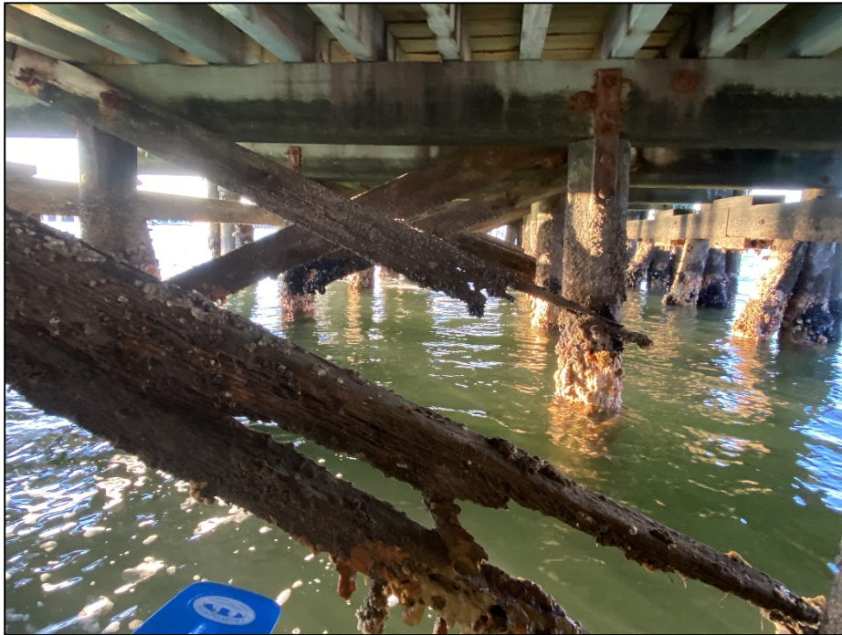
Photo No. 5.: Typical deterioration found below high water.
