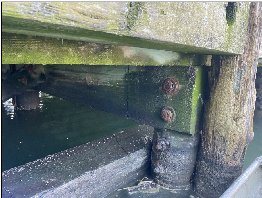
Photo No. 6.: Deterioration along pile caps.
