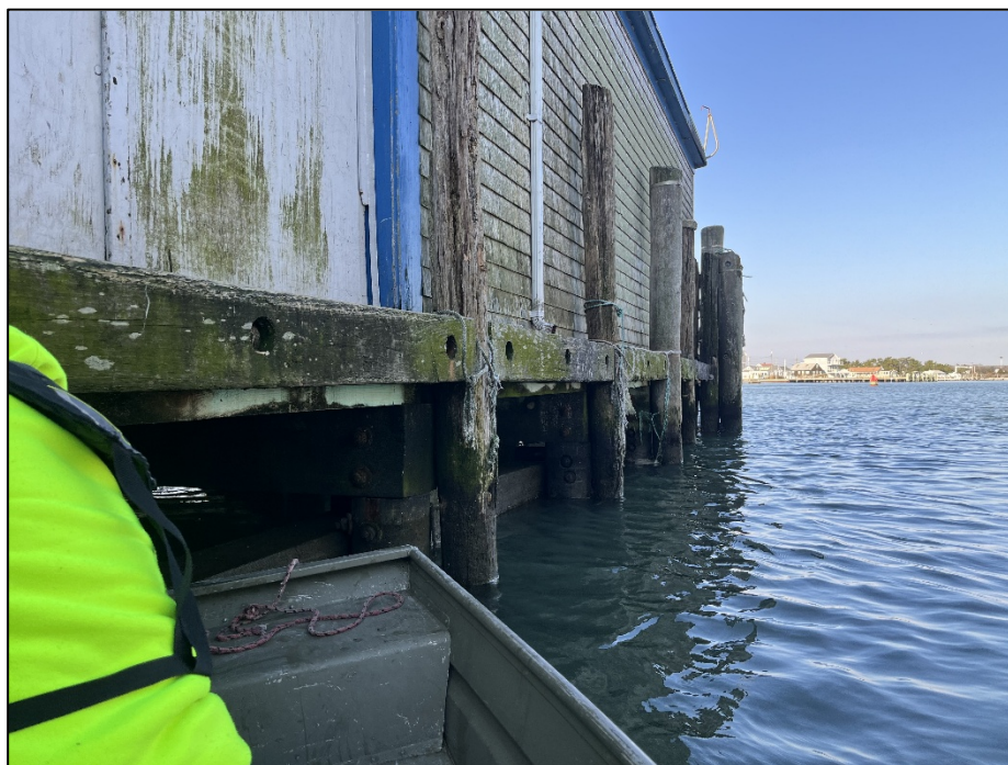
Photo No. 4.: Damage on fender piles due to limited ability of maintenance.
